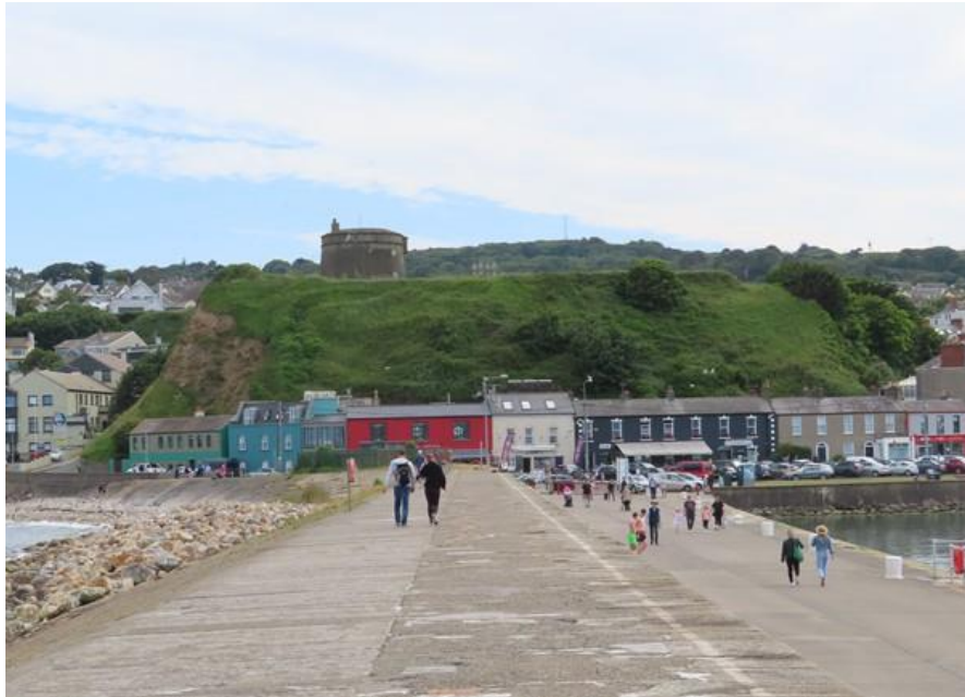
Plate 12 : View of Martello tower from landward end of East Pier
