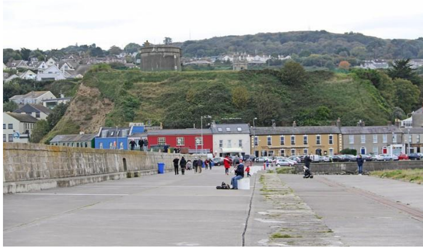
Plate 14: View of Martello tower from East Pier
