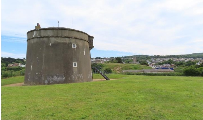
Plate 11: View southwards past tower towards application site
