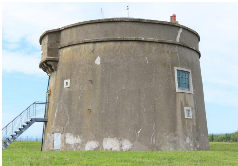
Plate 10 : Howth Martello tower seen from the east
